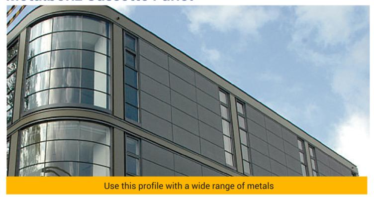
Metalbenz fabricates a panel with a recessed joint known as a 'cassette' panel. The left fold is indirectly fixed to the metal substrate with clips and the right recessed fold is married/overlapped to the next left side of the panel and fixed again with concealed clips.
